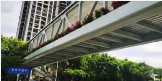
Photo: Community footbridge, Huizhou, China.
